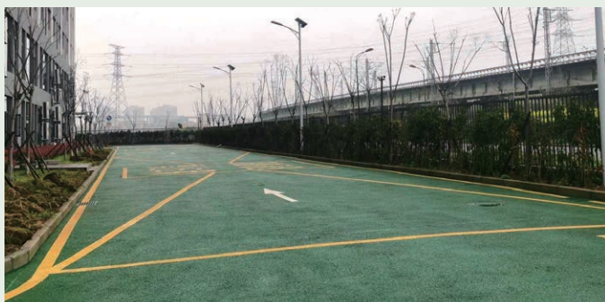
Permeable Concrete Construction in Hangzhou Park
